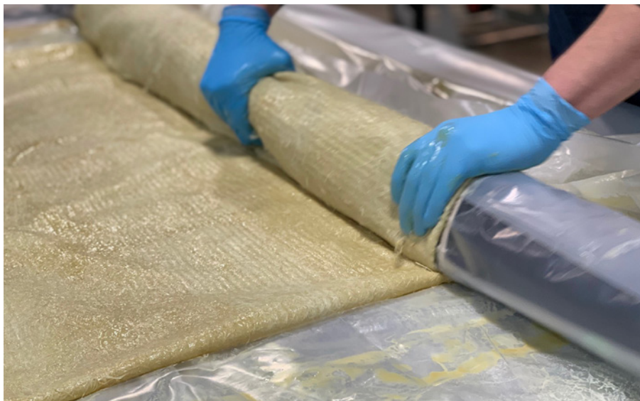
Fig. 9 Roll the resin-infused fibreglass around the polythene-covered lateral packer.
