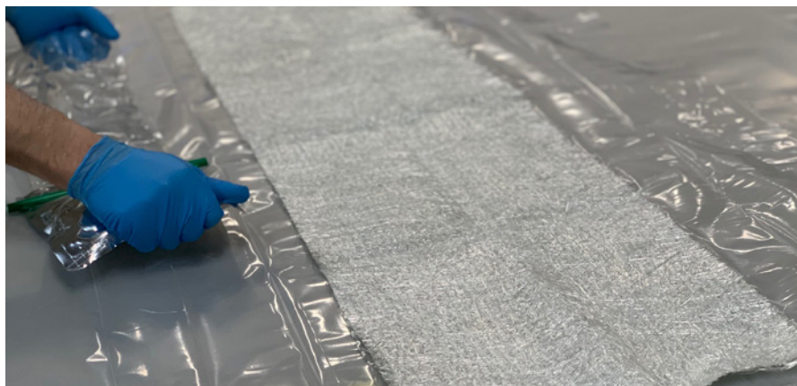
Fig. 3 Lay out the fibreglass sheets ready for the application of the resin.
