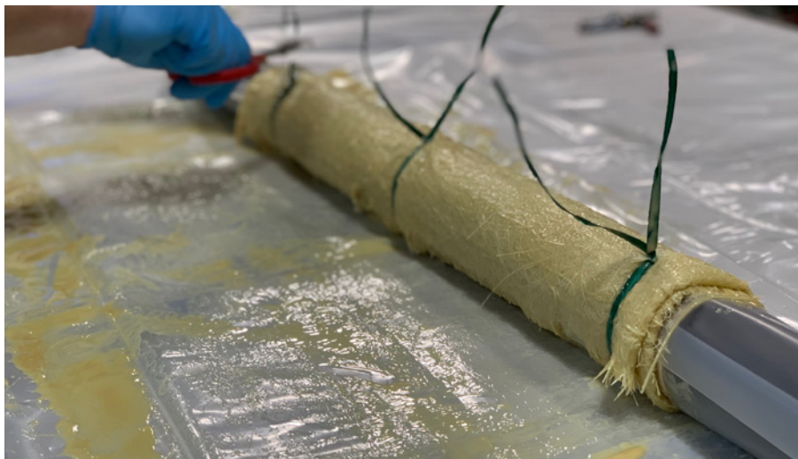
Fig. 10 Secure the resin-infused fibreglass using the supplied tie wraps, cut off the excess tie material after securing.
