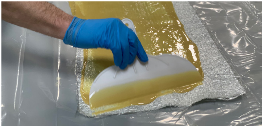
Fig. 6 Pour the well-mixed resin onto the fibreglass matting and spread out evenly.
