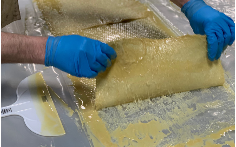
Fig. 7 Ensure that the resin is well mixed with the fibreglass and lift it as one piece.
