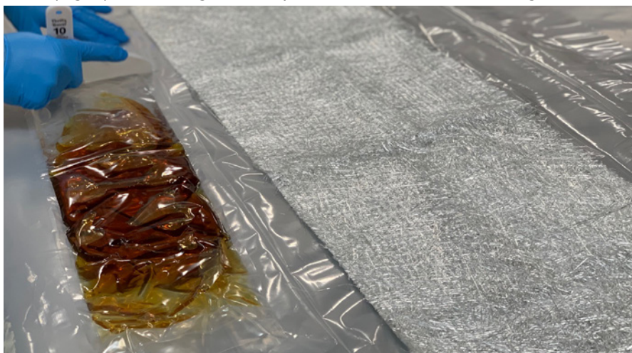
Fig. 5 Activate your resin pack and massage it from the outside for at least one minute to ensure that it is fully mixed.
