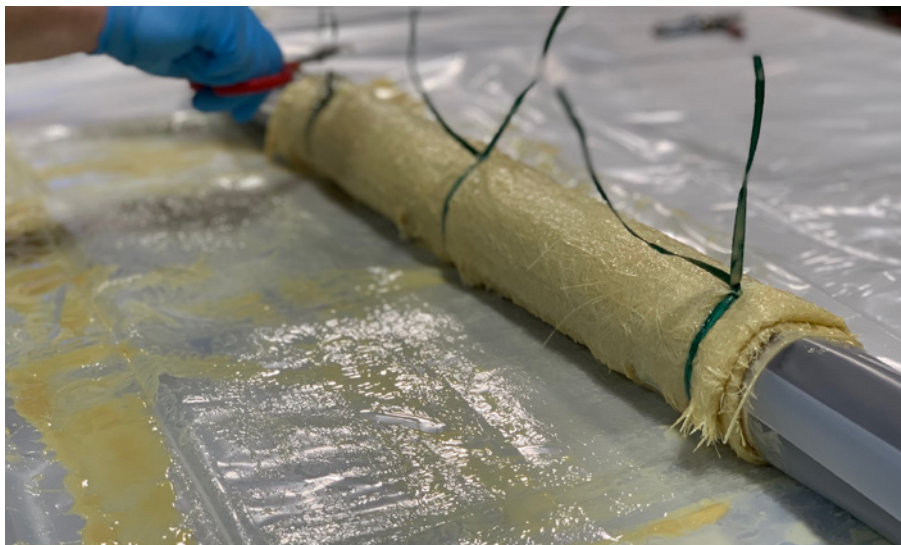
Fig. 10 Secure the resin-infused fibreglass using the supplied tie wraps, cut off the excess tie material after securing.
