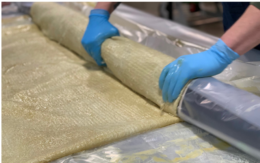
Fig. 9 Roll the resin-infused fibreglass around the polythene-covered flexible packer.
