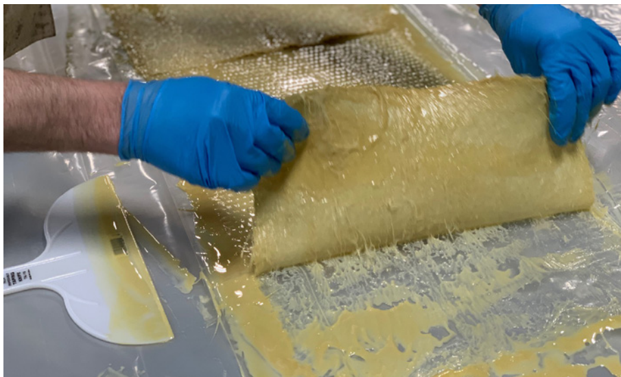
Fig. 7 Ensure that the resin is well mixed with the fibreglass and lift it as one piece.
