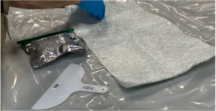
Fig. 2 Unpack the fibreglass sheets and resin bags and necessary tools.
